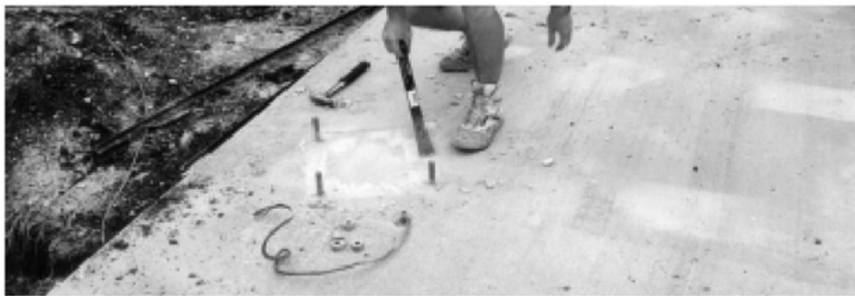
Figure 1-2: Scraping Foundation Pads
