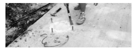
Figure 1-3: Scraping Foundation Pads
