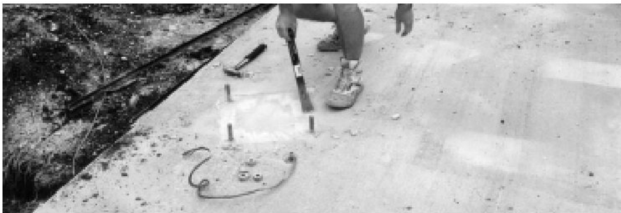
Figure 1-3: Scraping Foundation Pads
