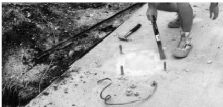
Figure 1-3: Scraping Foundation Pads
