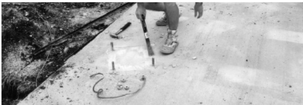
Figure 1-3: Scraping Foundation Pads
