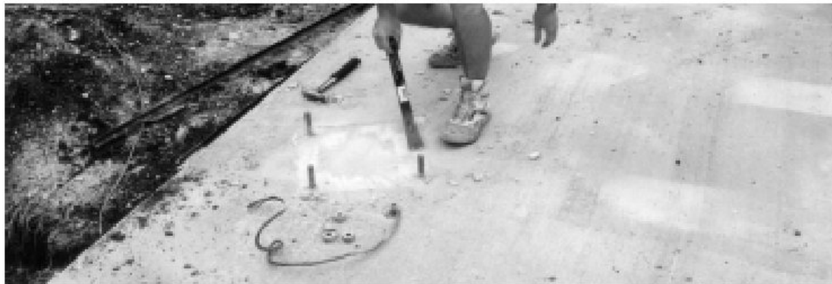
Figure 1–2: Scraping Foundation Pads
