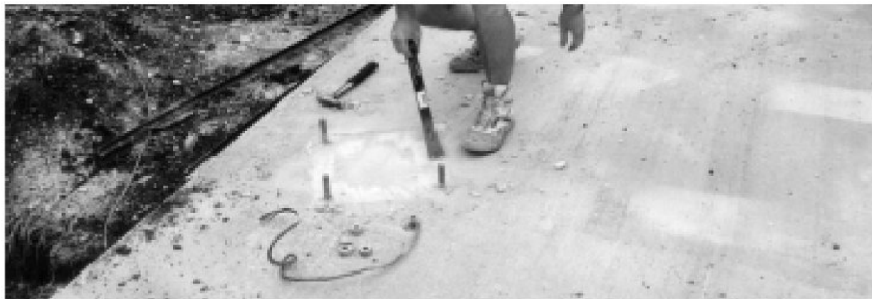
Figure 1-2: Scraping Foundation Pads
