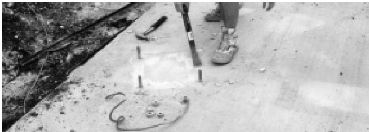
Figure 1-3: Scraping Foundation Pads
