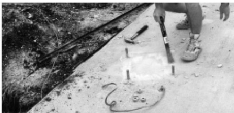
Figure 1-3: Scraping Foundation Pads
