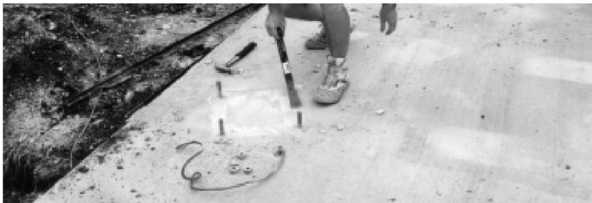
Figure 1-2: Scraping Foundation Pads
