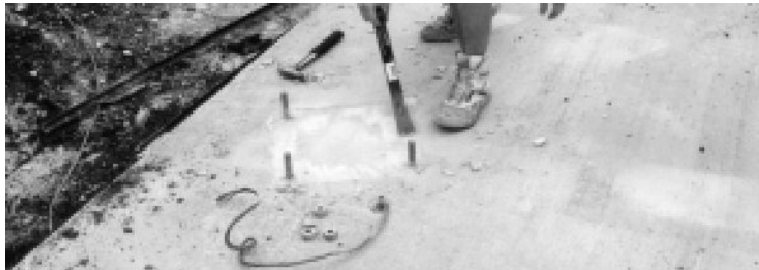
Figure 1-3: Scraping Foundation Pads
