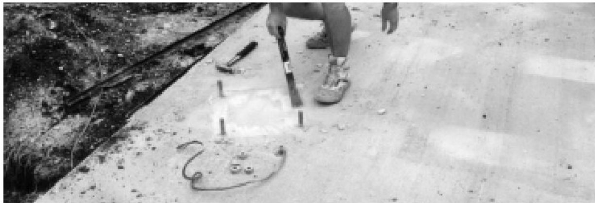
Figure 1-2: Scraping Foundation Pads
