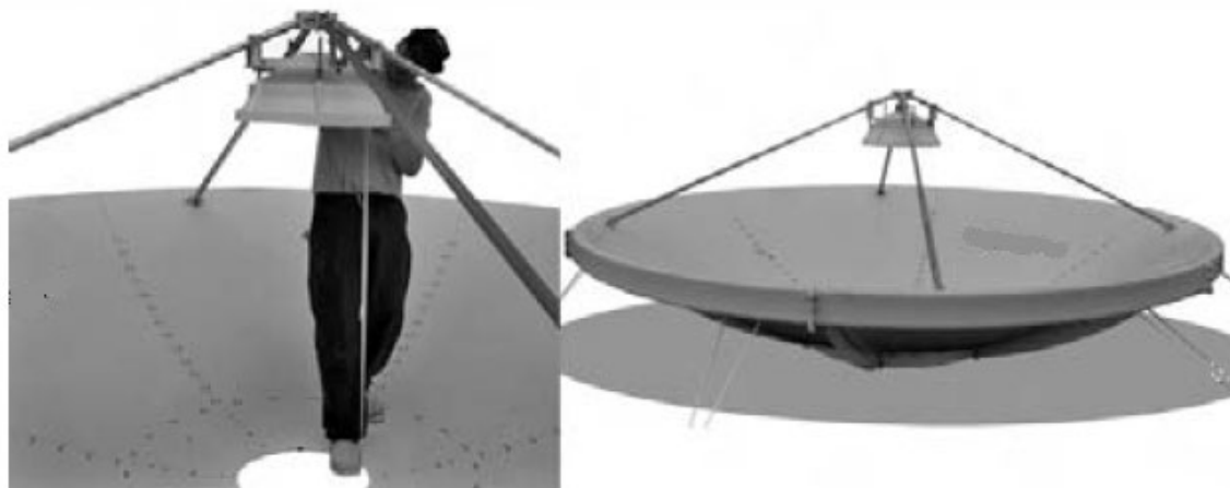
Figure 82 – Subreflector Adjustment
